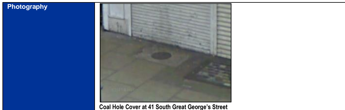
Coal Hole Cover at 41 South Great George's Street
